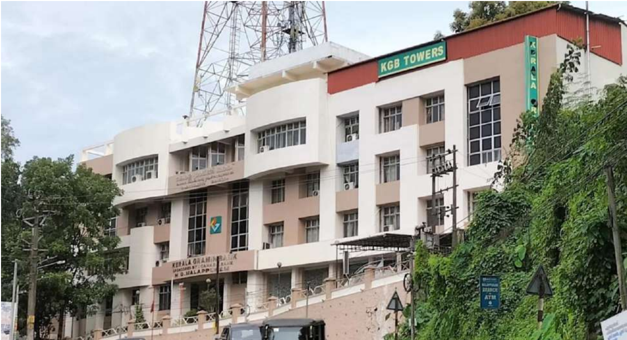
EXISTING FRONT FAÇADE OF KGB HO BUILDING
